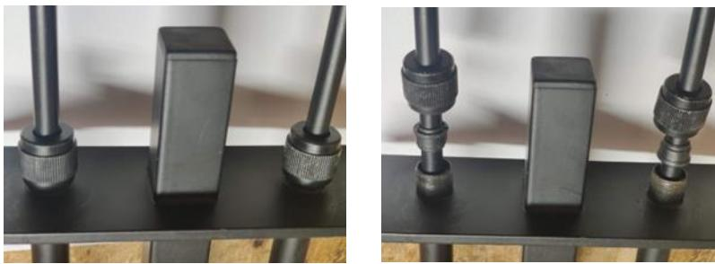
Loosen the 2 clamp nuts on the black suspension rods and hang the fixture at the correct height. Tighten these nuts securely.
